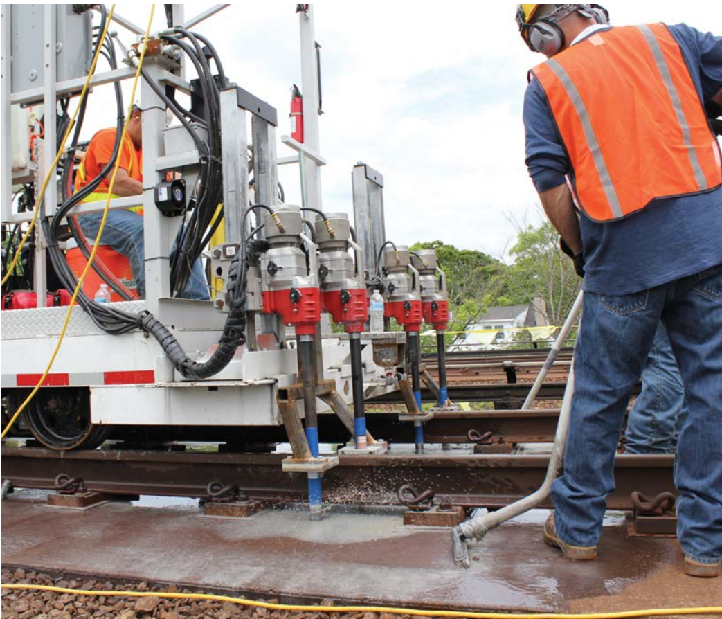
Slurry created during the drilling work was controlled by wet vacuums.
